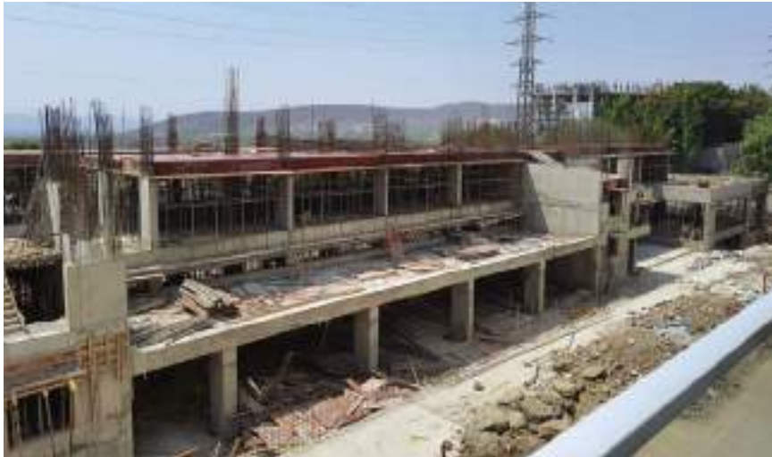
VJ HAPPINESS STREET- 4 TH SLAB SHUTTERING & REINFORCEMENT WORK IS IN PROGRESS.
