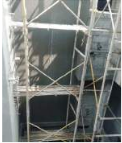
YASHWIN ENCORE - 'B1B2' PLASTER WORK IS IN PROGRESS IN DUCT AREA.
